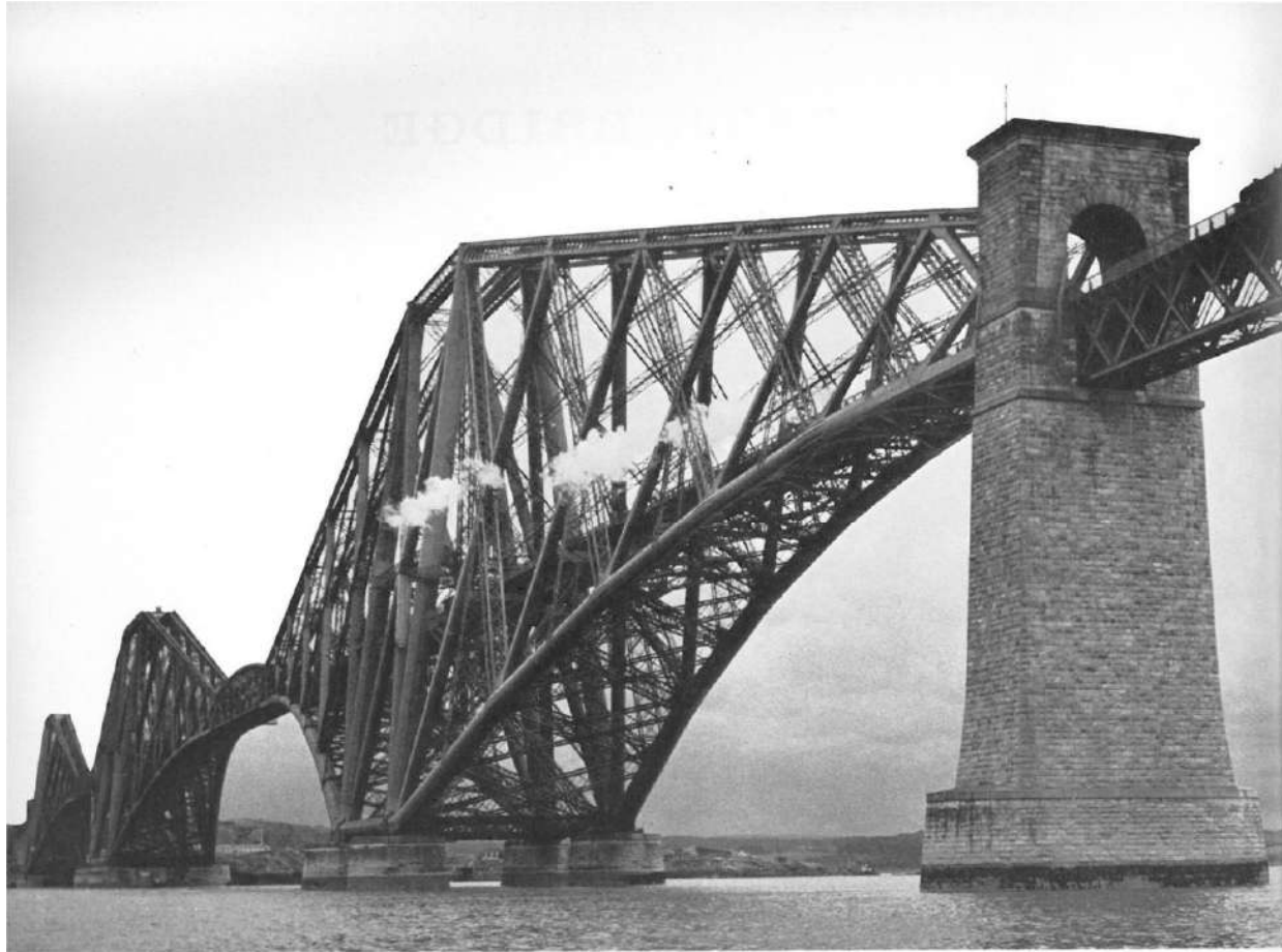
The three cantilever towers of the Forth Bridge, with one of the massive piers which form the abutments for the shore cantilever arms. On the extreme right can be seen the locomotive of a train about to cross the bridge.
